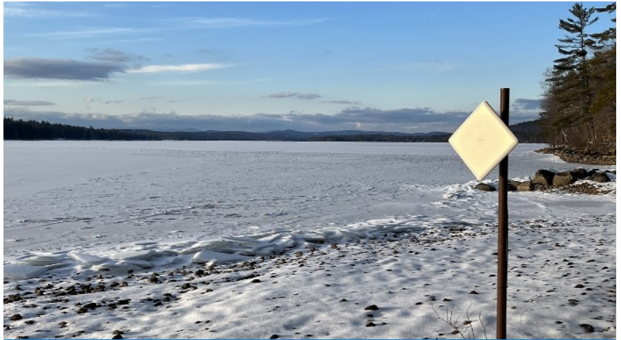
BEC RidgeWave® 6900R21 CBRS outdoor router is installed at a residence along Long Lake in Harrison, ME by Outer Reach Broadband in January 2022.
